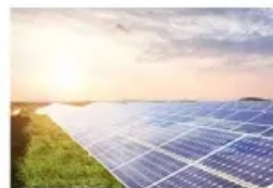
Energy Storage System
