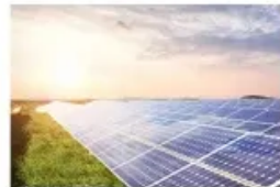
Energy Storage System
